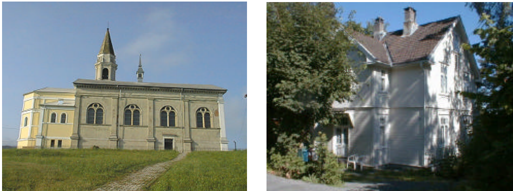
Figure 5: A retrofitted church building in Slovenia, equipped with a wall tempering system, and a wooden residential building in Norway, equipped with advanced waterborne floor, wall and ceiling heating systems (Annex 37 2004).
